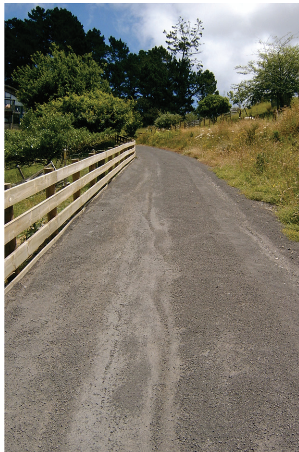
Driveway with MetalMaxx® used for surfacing
