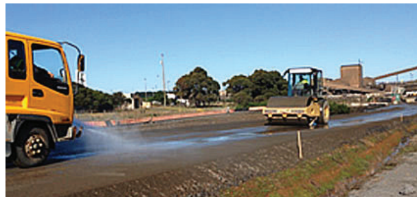
Compaction Roller following a water cart.
